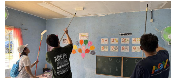
Daycare centre renovation in the Philippines
